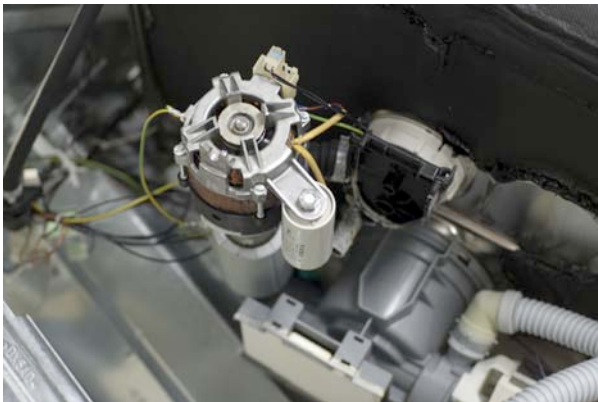
Inlet pump and motor
